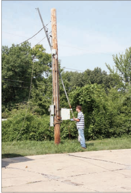
Technician performing maintenance/calibration at the site. All microphones are on tilt down poles for easy access during calibration.
