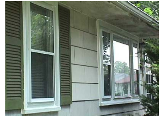
Structure after window treatment
