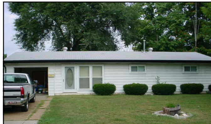
Completed structure with new door and windows
