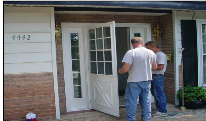
Acoustical storm door being installed
