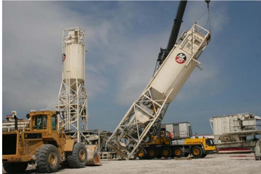
A portable batch plant is erected at Lambert this week.
