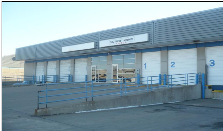
Image: Cargo Building 4. Photograph taken on 2/5/09.
