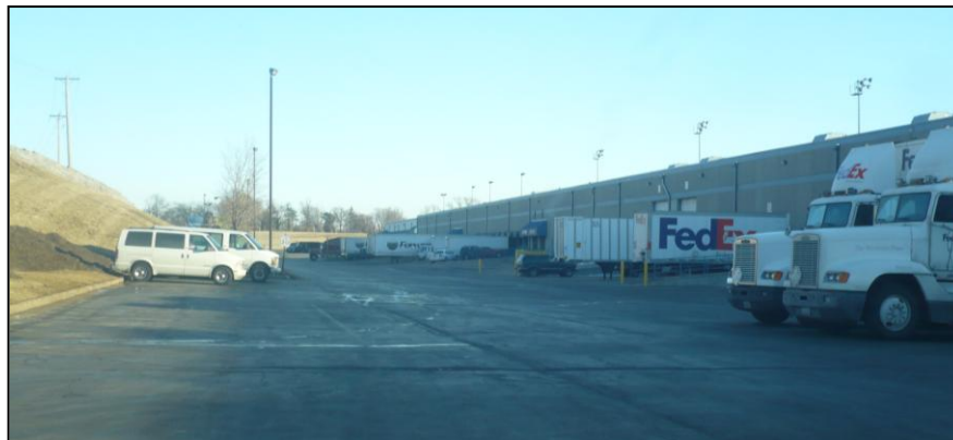
Image: Truck loading area of Commercial Air Cargo Facility, looking southeast. Photograph taken on 2/5/09.
