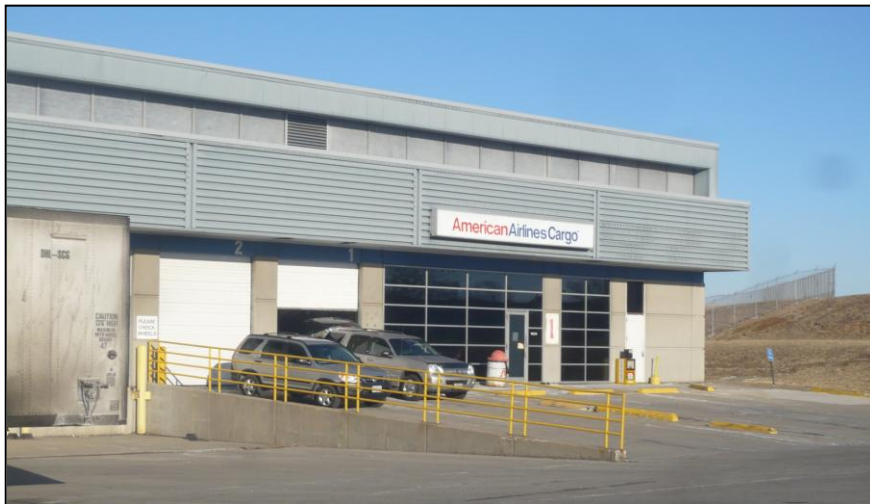
Image: American Airlines Cargo Facility in Cargo Building 1. Photograph taken on 2/5/09.
