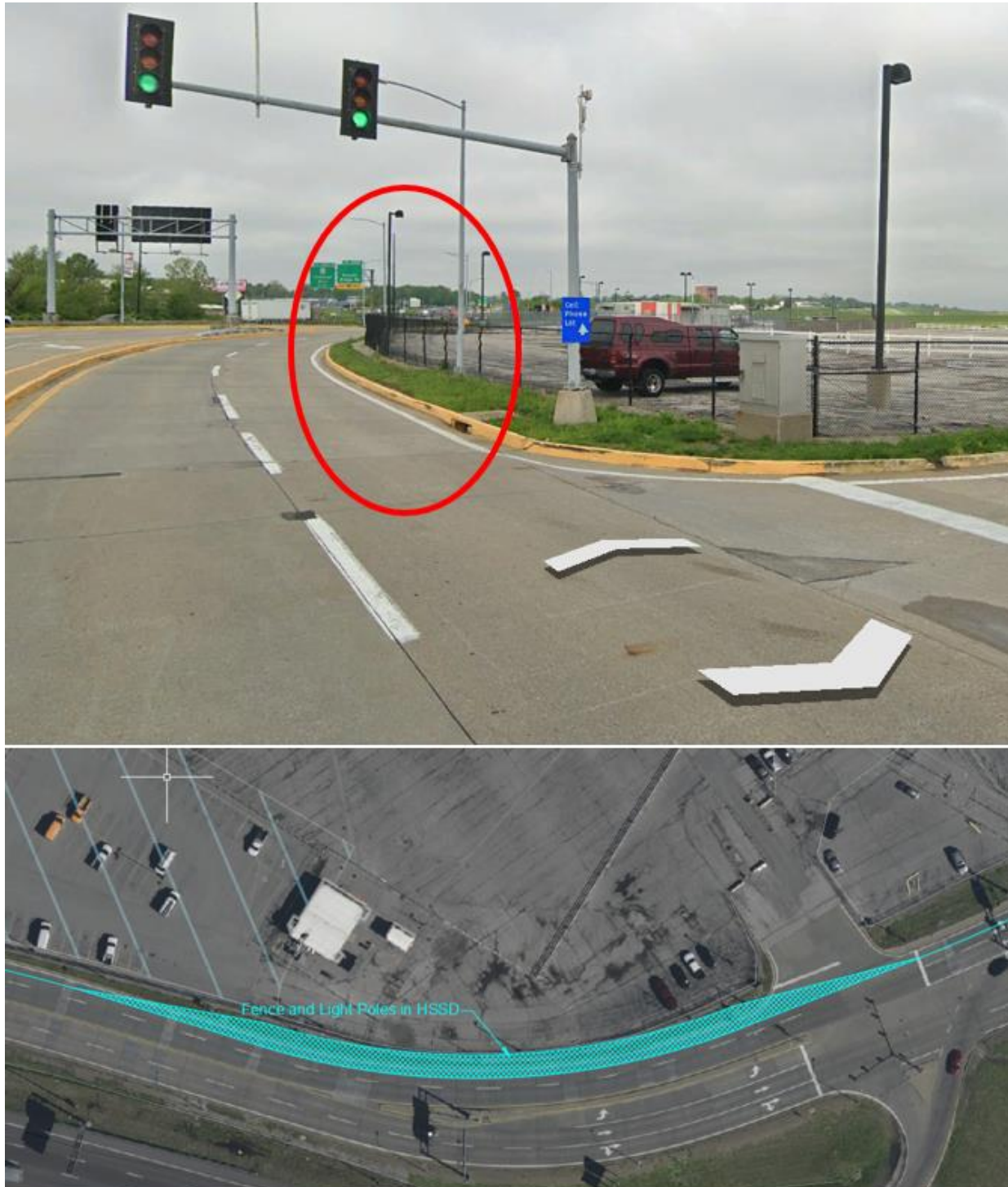
Figure 4.3-4: Insufficient Horizontal Sight Distance on Lambert International Blvd
