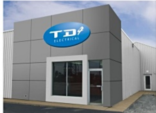
TD4 Electrical Headquarters
