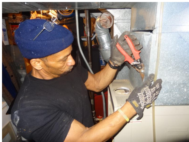
Mike Harris with Williams Heating and Cooling repairs homeowner's furnace.
