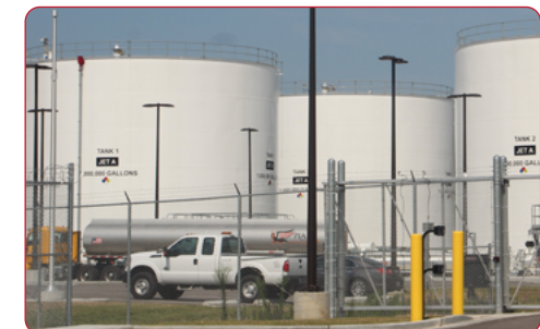
STL's New Fuel Farm Facility
