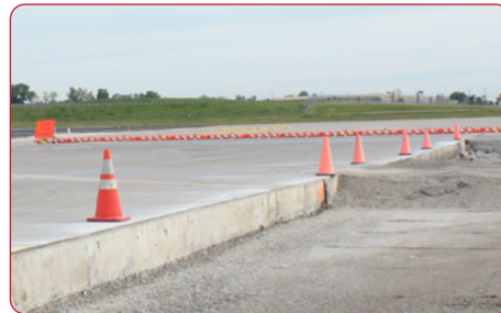
Reconstruction of Taxiway Delta
