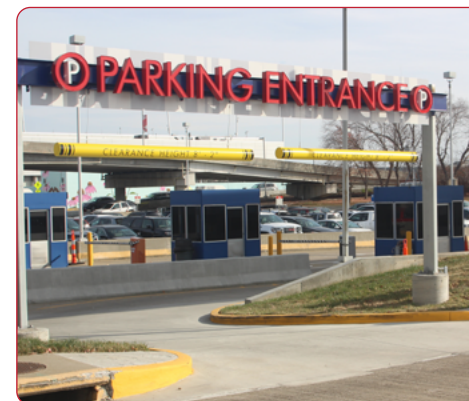
New Westbound Entrance of T2 Garage
