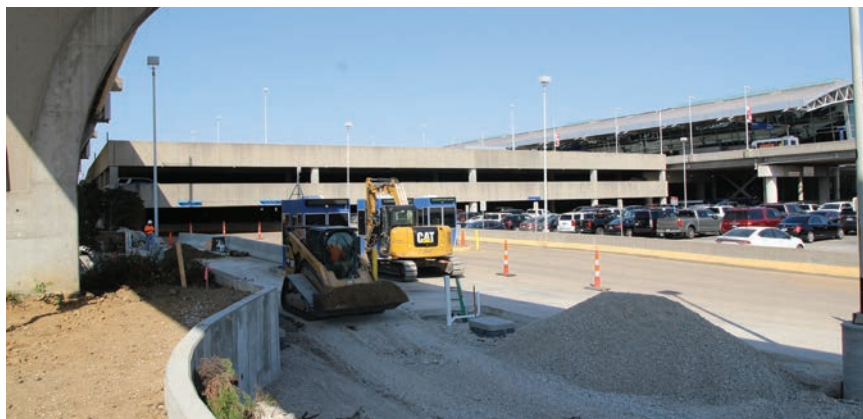
Terminal 2 Road and Garage Construction
