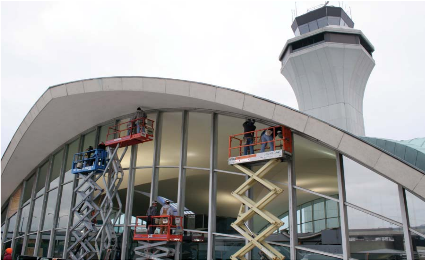
Four lifts were used to install new windows in Terminal 1 this week.
