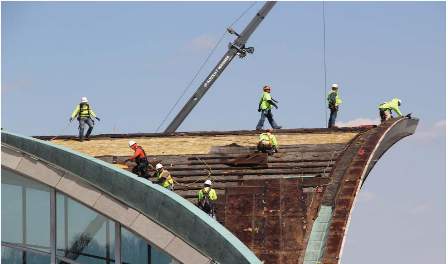
Roofing crews began the demolition of Lambert's 60 year old copper roof this week.
