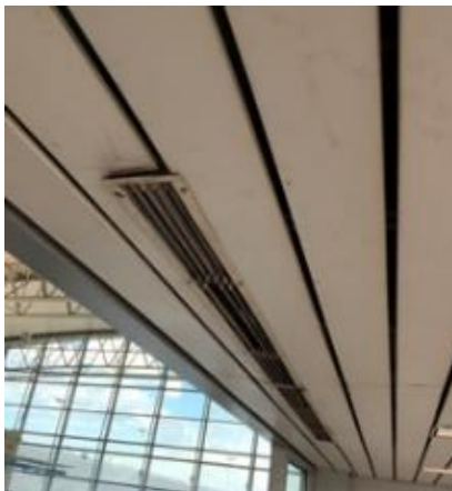
Figure 11.2-2: Representative Door Air Curtain in Terminal Entrance
