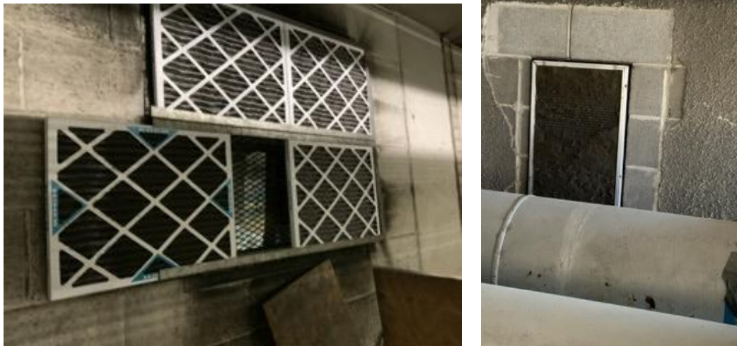
Figure 11.2-3: Fouled Air Filters Inhibiting Air Flow
