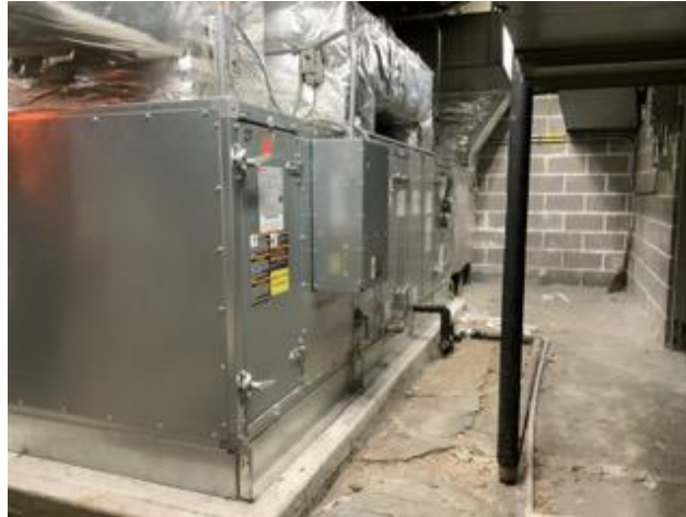
Figure 11.2-13: Typical Newer Indoor Modular Air Handling Unit
