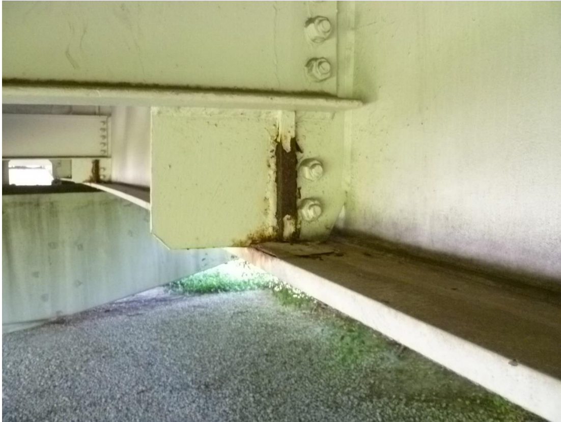
Figure 11.2-37: Rusted intermediate diaphragm connector plate on Departures Drive Bridge
