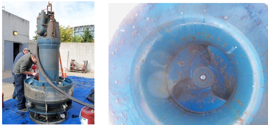
Figure 11.2-42: Primary Stormwater Pumps and Impeller (Per Previous Inspection by Others)
