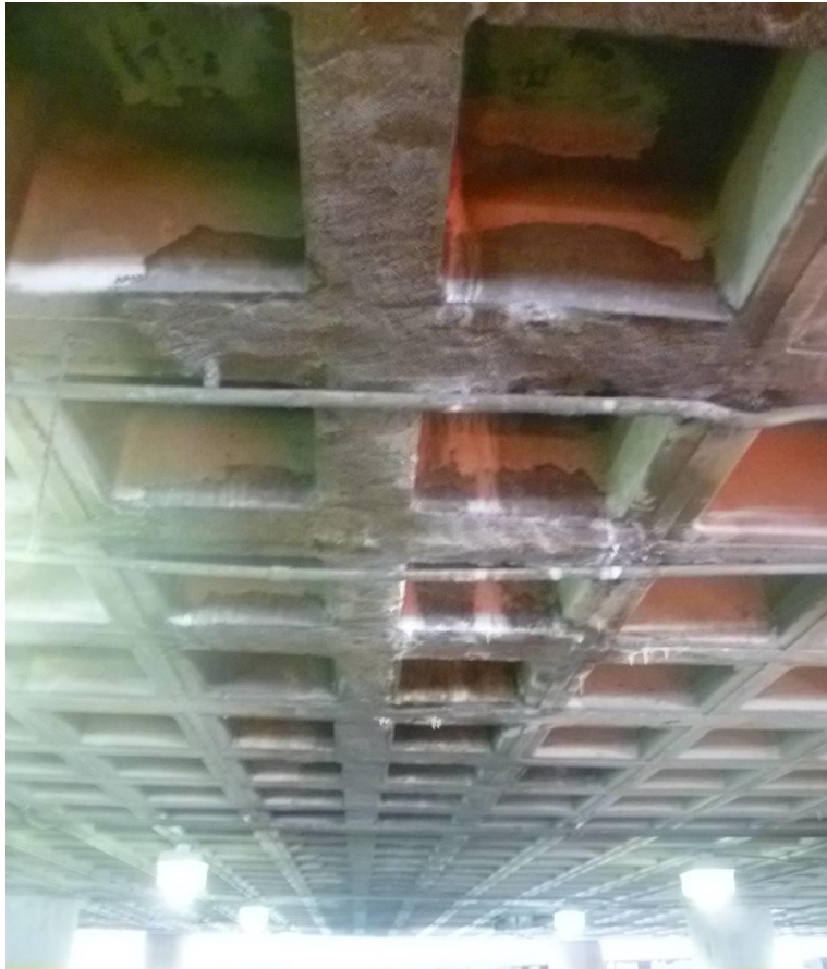
Figure 11.2-30: Arrivals Drive Bridge Slab (underside) showing previous patches and efflorescence
