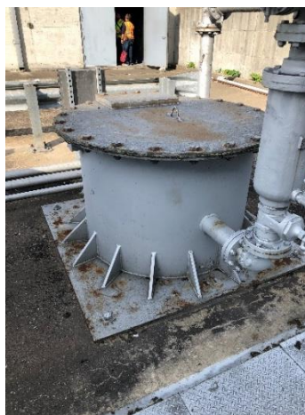
Figure 11.2-43: Example of a Primary Stormwater Pump Housing and Valve
