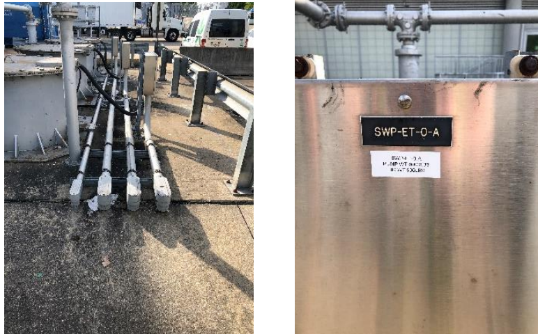
Figure 11.2-44: Electrical Conduit and Control Panels
