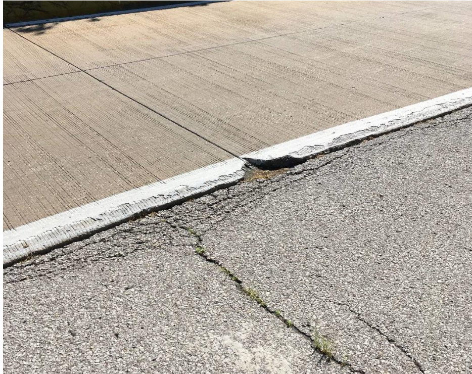
Figure 11.2-31: Pavement and shoulder deterioration typical of Ramps A and D approaches
