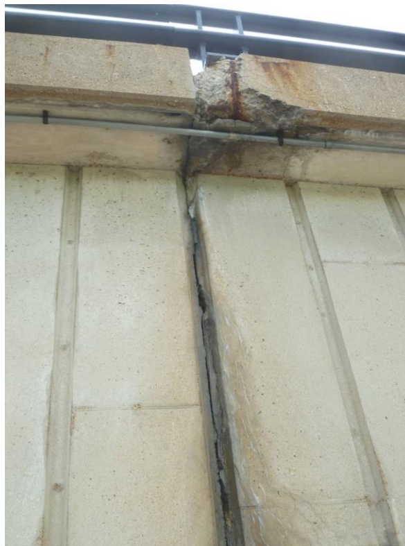
Figure 11.2-39: LIB over Airflight Drive Bridge approach retaining wall joint and barrier curb showing significant deterioration
