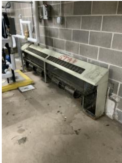
Figure 11.2-14: Fan-Coil Unit Representative of Apron Level Terminal Equipment
