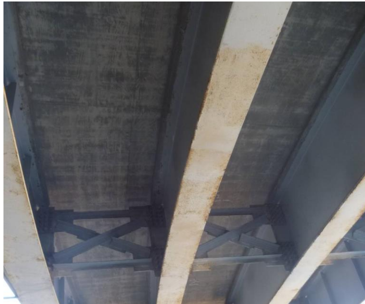
Figure 11.2-33: Bottom of Ramp D girders showing deterioration of paint
