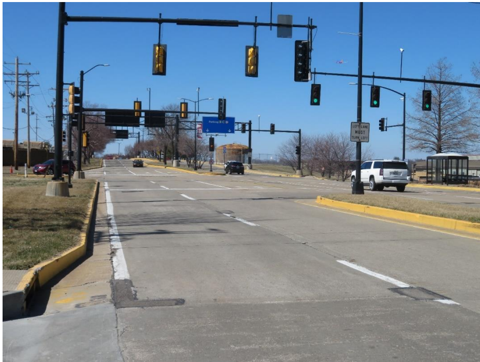
Figure 11.2-38: LIB showing typical pavement patching and worn curbs
