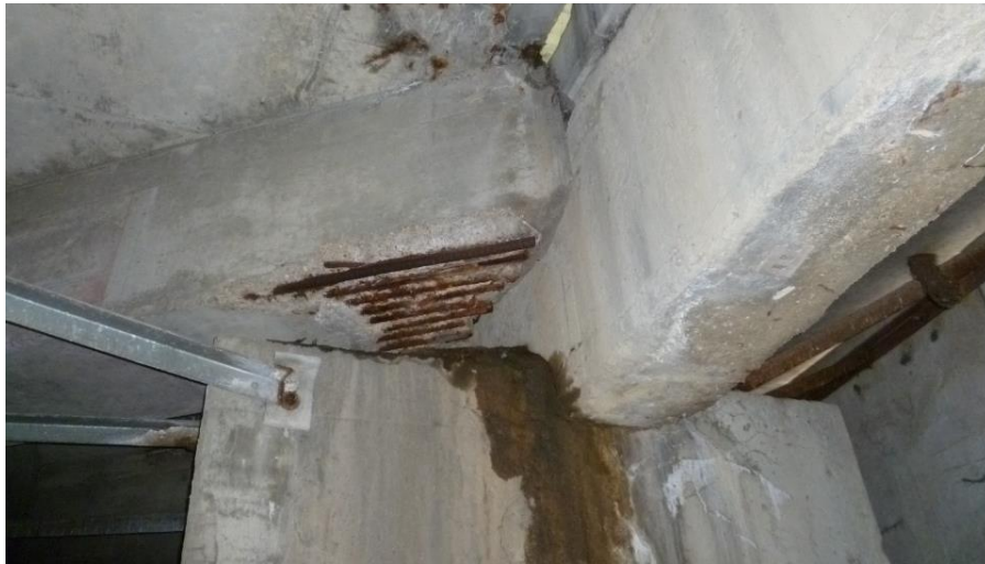
Figure 11.2-35: Departures Drive over Arrivals Drive Bridge – Deteriorated beam ends and water leakage within area enclosed by fascia panels
