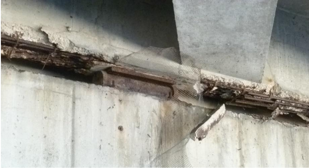
Figure 11.2-34: Departures Drive over Arrivals Drive Bridge southwest end beam showing deteriorated concrete, exposed rebar, and rusted bearings
