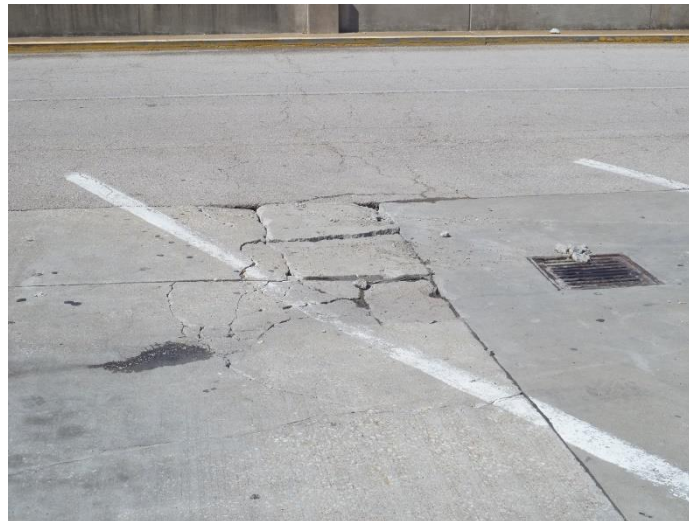
Figure 11.2-32: Departures Drive showing deteriorated driving surface
