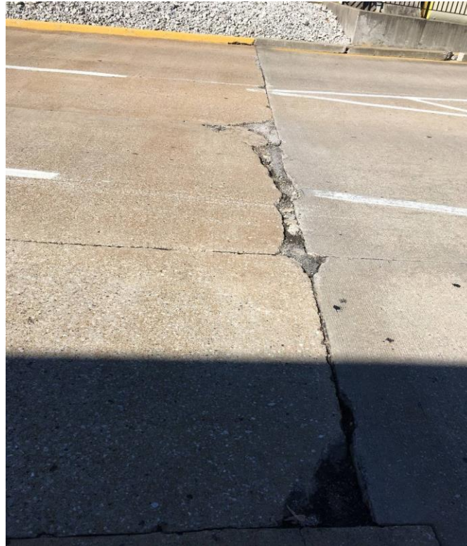
Figure 11.2-29: Arrivals Drive – Deteriorated Pavement and Curb
