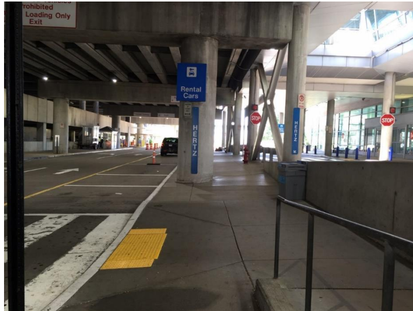
Figure 11.2-36: Non-reflective signage and worn pavement markings on Arrivals Drive
