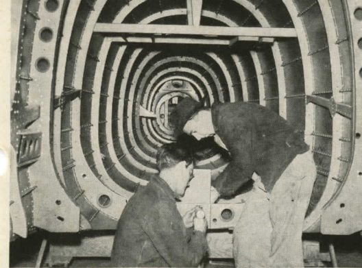
Bulkheads and Stringers—The Belly of the AT-9.
